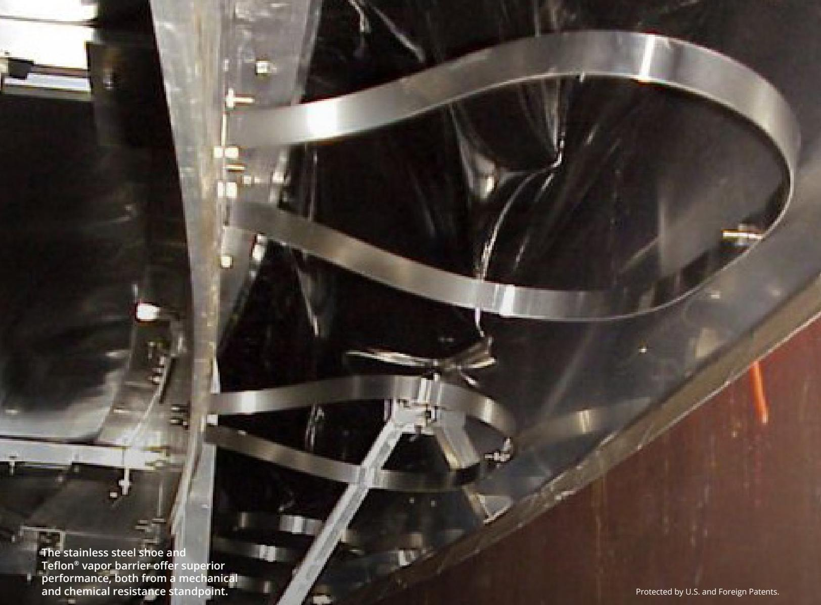
The stainless steel shoe and Teflon® vapor barrier offer superior performance, both from a mechanical and chemical resistance standpoint.
